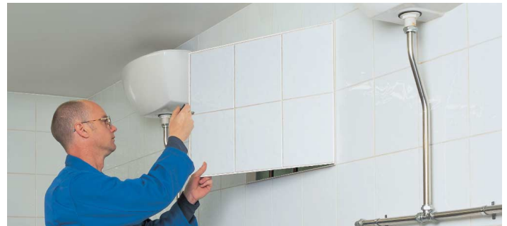
FIG 3 ELEVATION TILED WALL DOOR, BUDGET LOCK OPERATED
